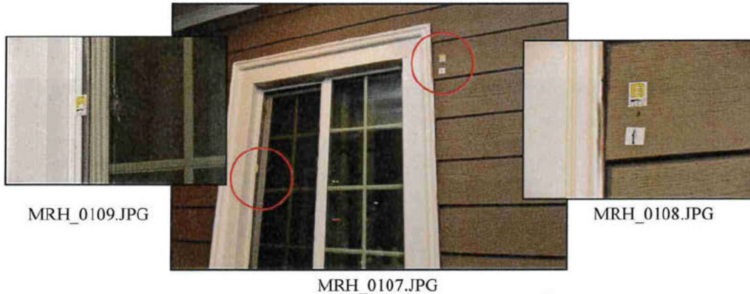
Figure #5: Two defects caused by bullets at [REDACTED]
